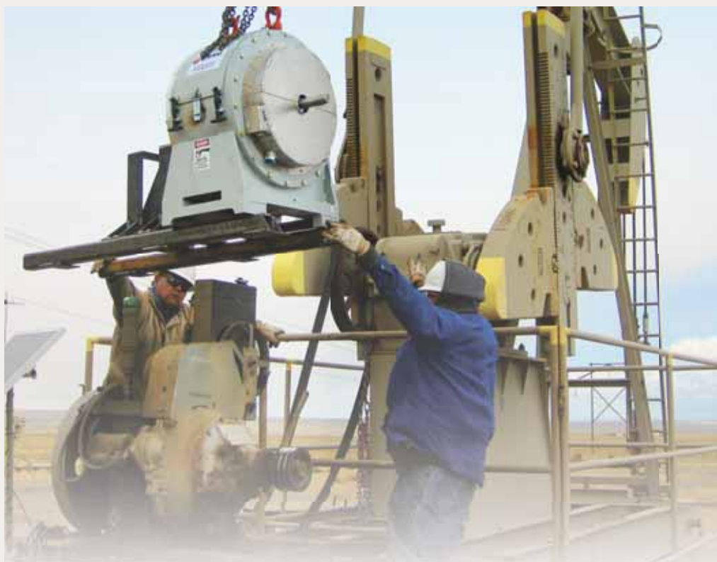
► Oil-field workers installing the transmission on a working natural gas well near Farmington, NM. The transmission is hanging on the hoist, and the engine is below and slightly to the left.
